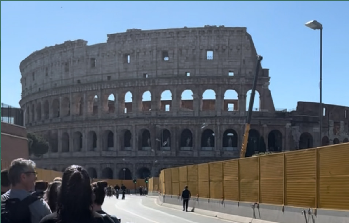
Construction work for the metro line near the Roman Colosseum, Italy. © RERM
